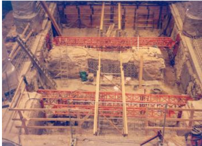
Fig. 12: Stutten schip
