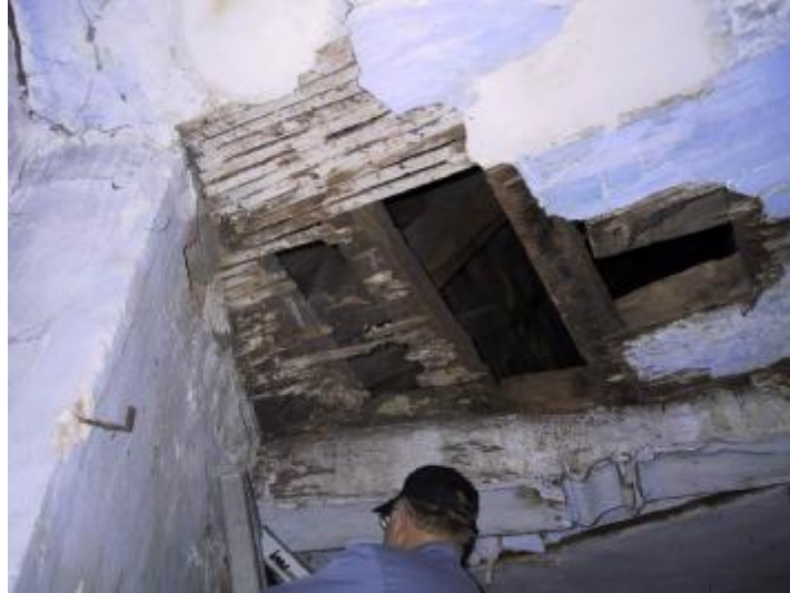
Fig. 11: Vochtaantasting houten roostering
