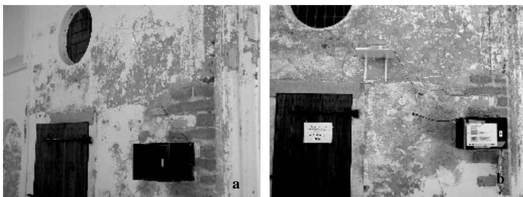
Fig. 12: Situation of the damage at Nov. 2001 (a) and at September 2004 (b): a clear increase of the damage is visible
