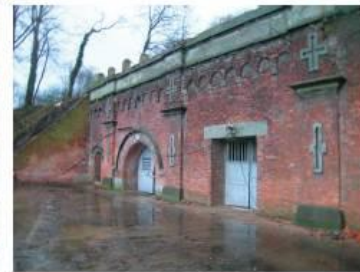
BAY 01 - BAY 02 - BAY 03 of RCAP 22.01.2005
