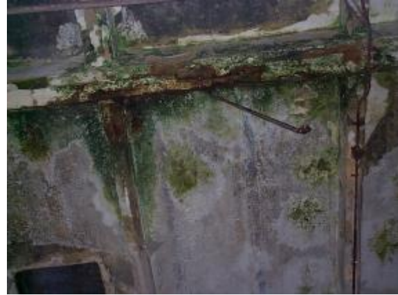
Fig. 4b: Moss growth on the structure
