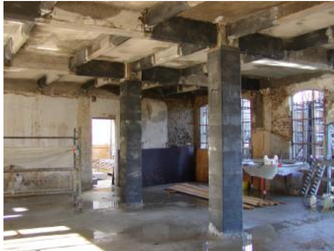
Fig. 15: Strengthened construction, on floor level 0
